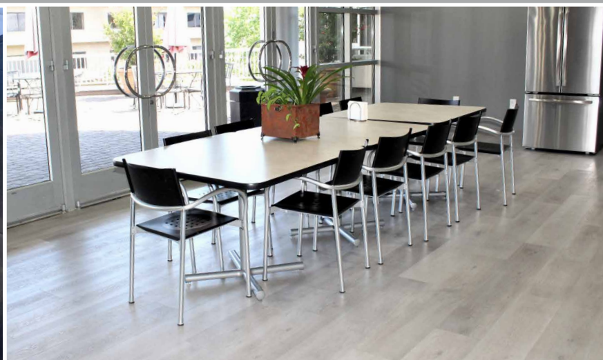
Attraxion installation over MagneBuild underlayment in process.
